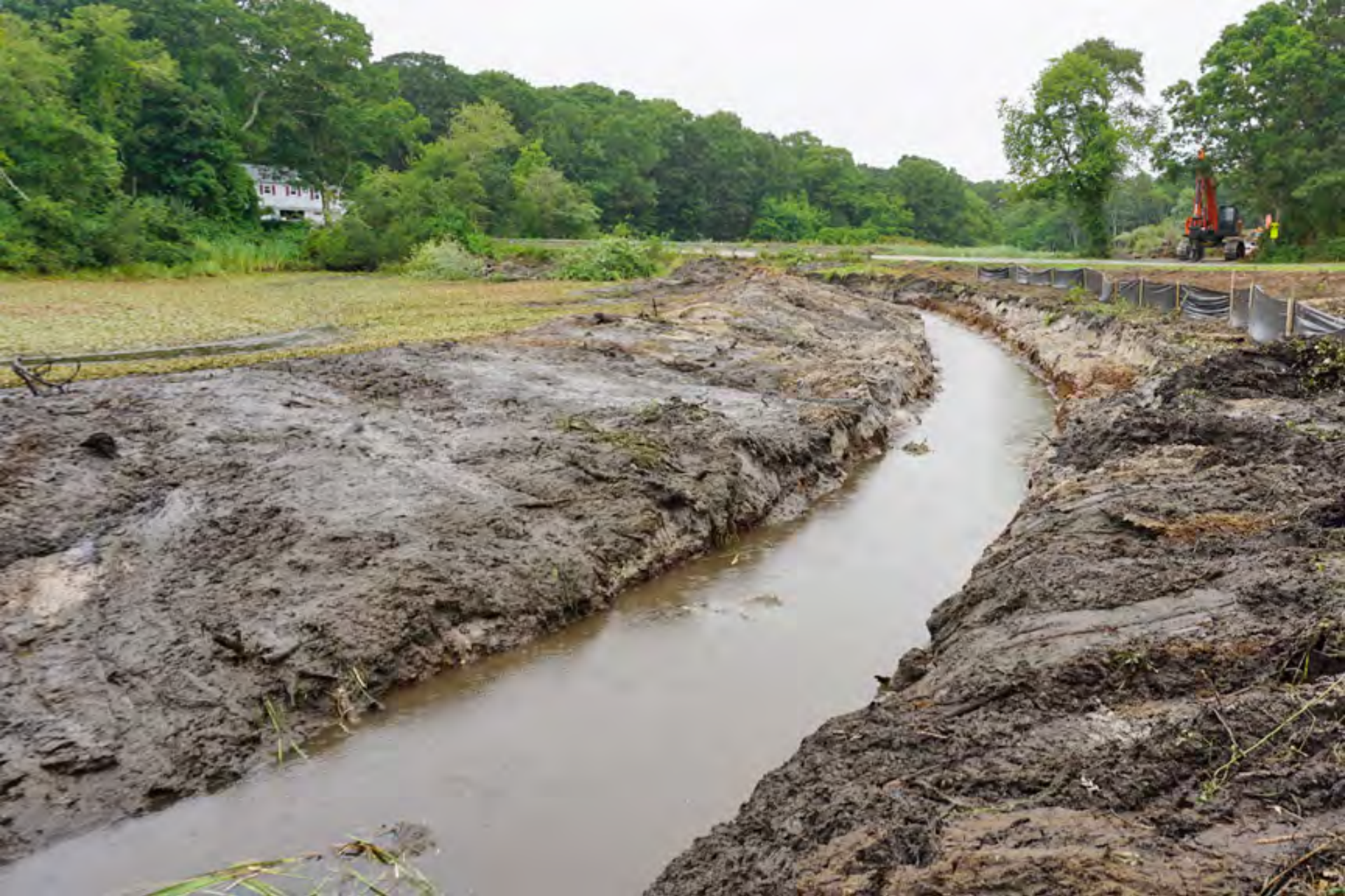
Bypass channel construction
