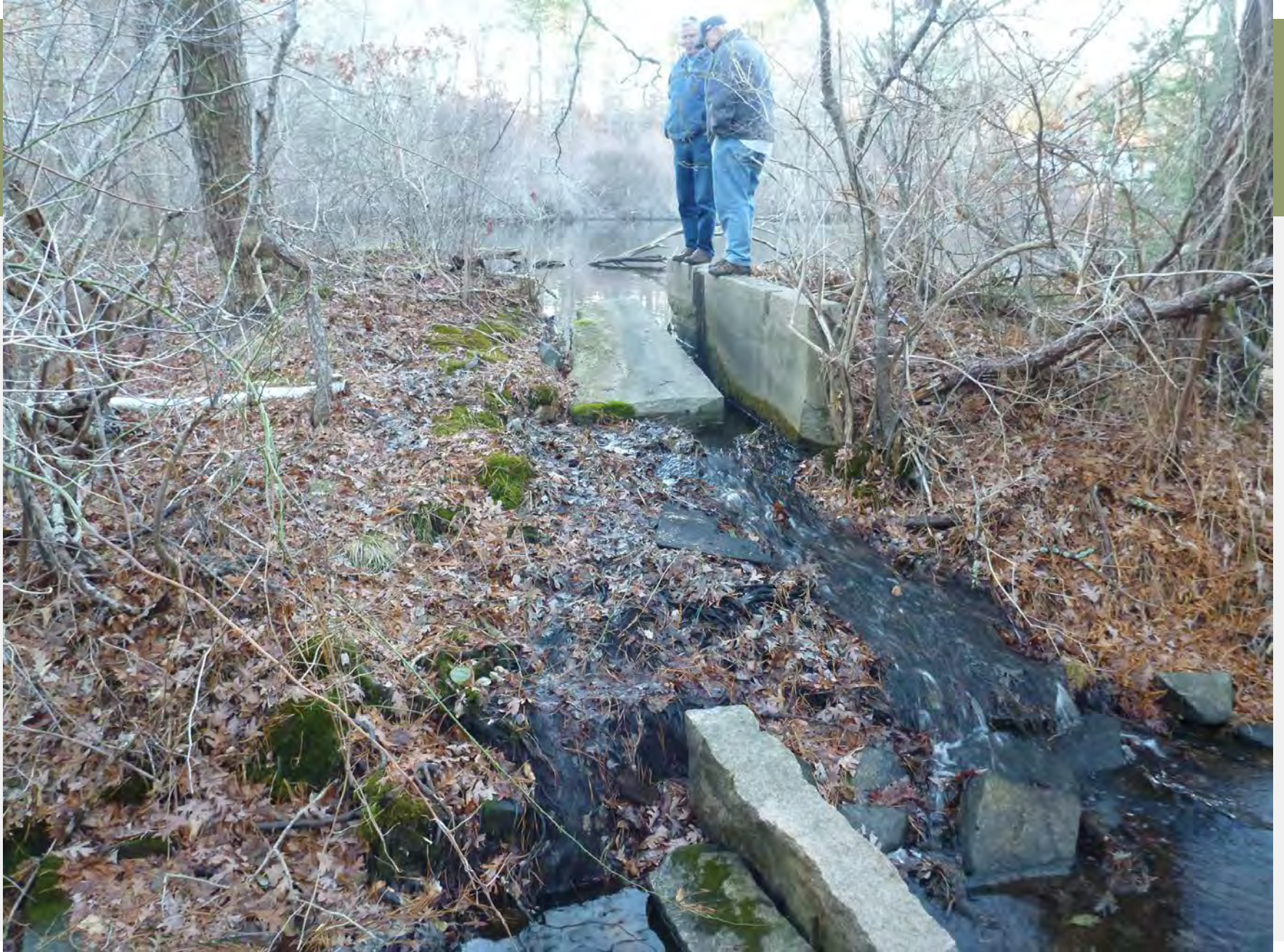
Earthen Dam Existing Conditions
