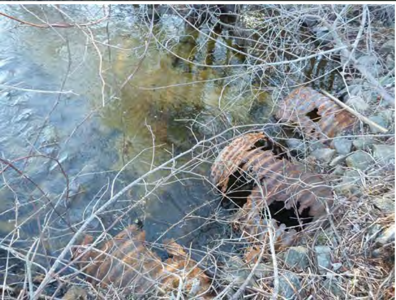
John Parker Road culverts, Falmouth, 2017
