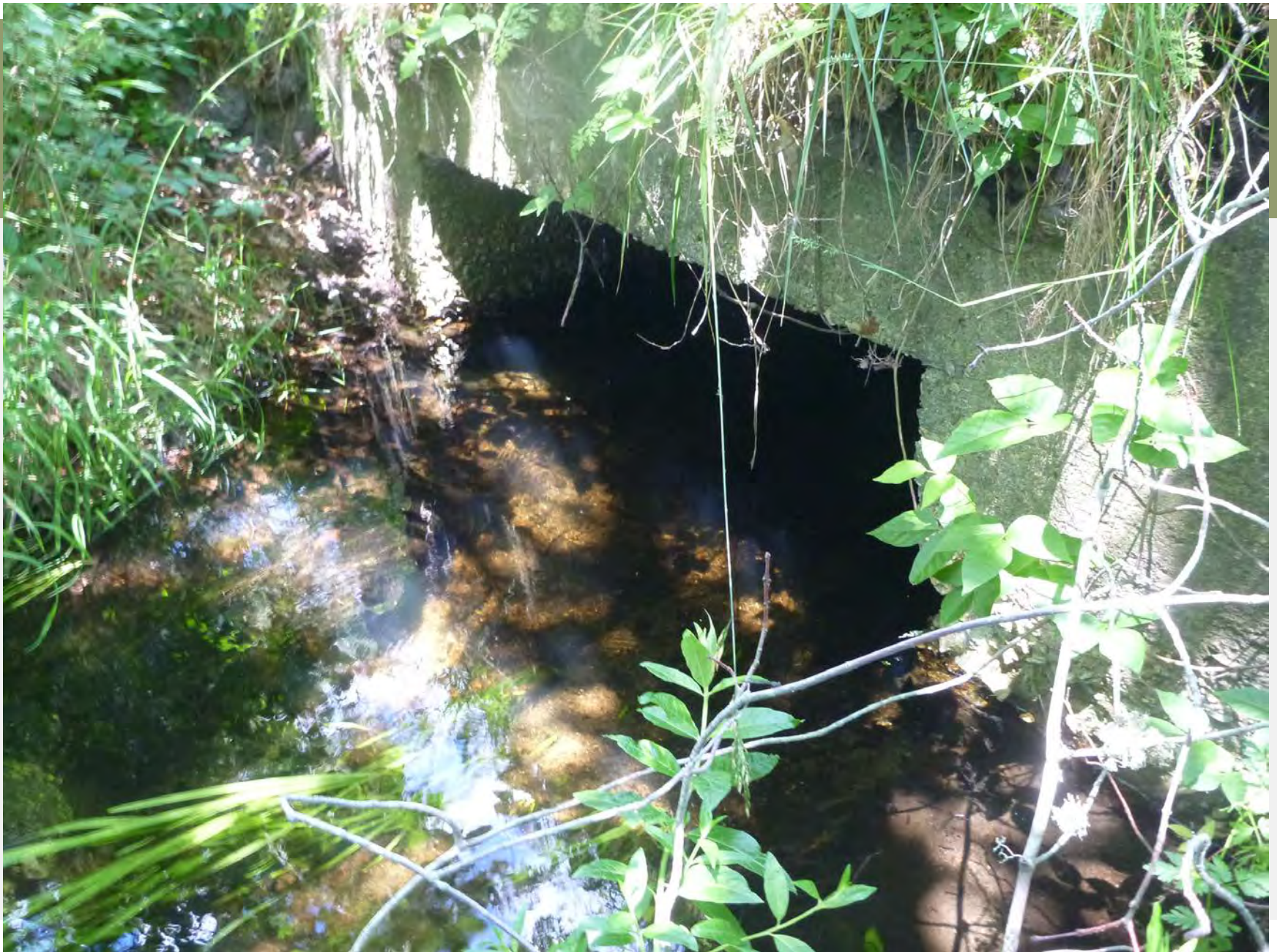
Carriage Shop Road Culvert Existing Conditions
