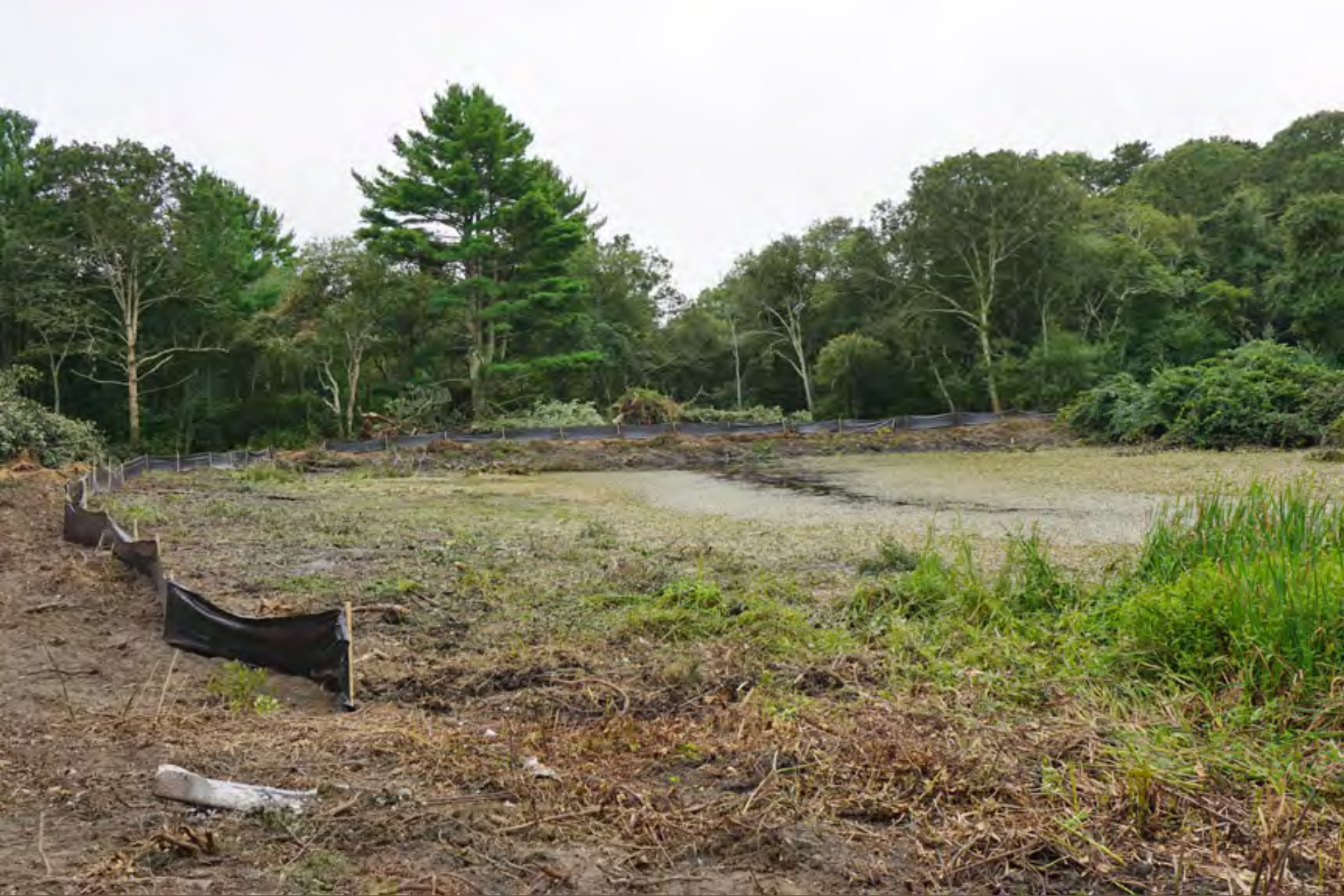
Dam notching and impoundment drawdown
