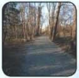
Stabilized Aggregate Multi-Use Path
